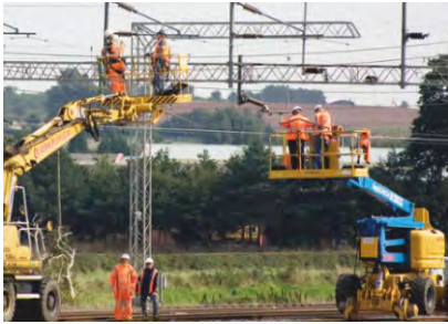
Overhead Line Maintenance
