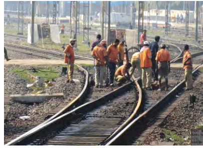
Maintenance of railway line without the gauge
