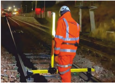
Measuring using the Live Line Gauge
